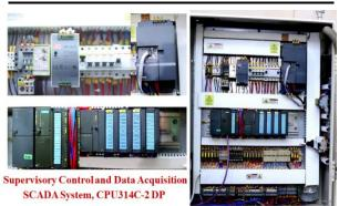
Figure 16: Second control panel components.
