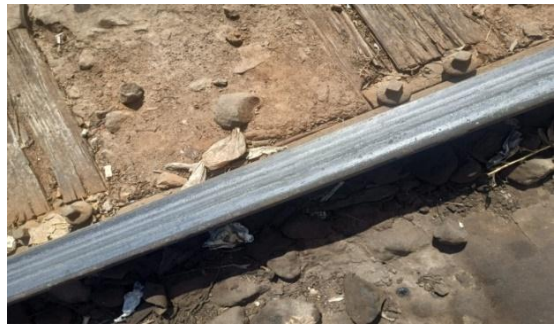
Figure 10: worn rail
