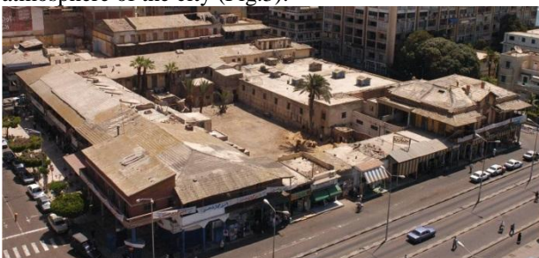
Figure 3: Current Condition of National Hotel Building.
