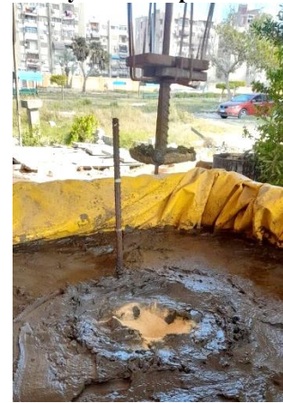
Figure 12: Weak layer surface after application of dynamic replacement with sand
