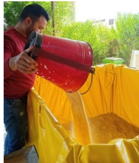
Figure 7: Adding a bottom layer of sand.
