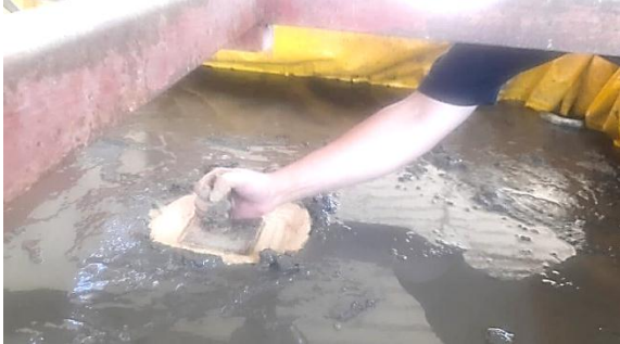
Figure 9: Preparation of partial replacement under footing
