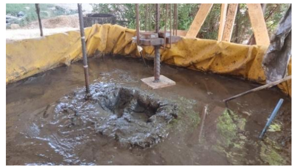
Figure 11: Weak layer surface after application of dynamic compaction
