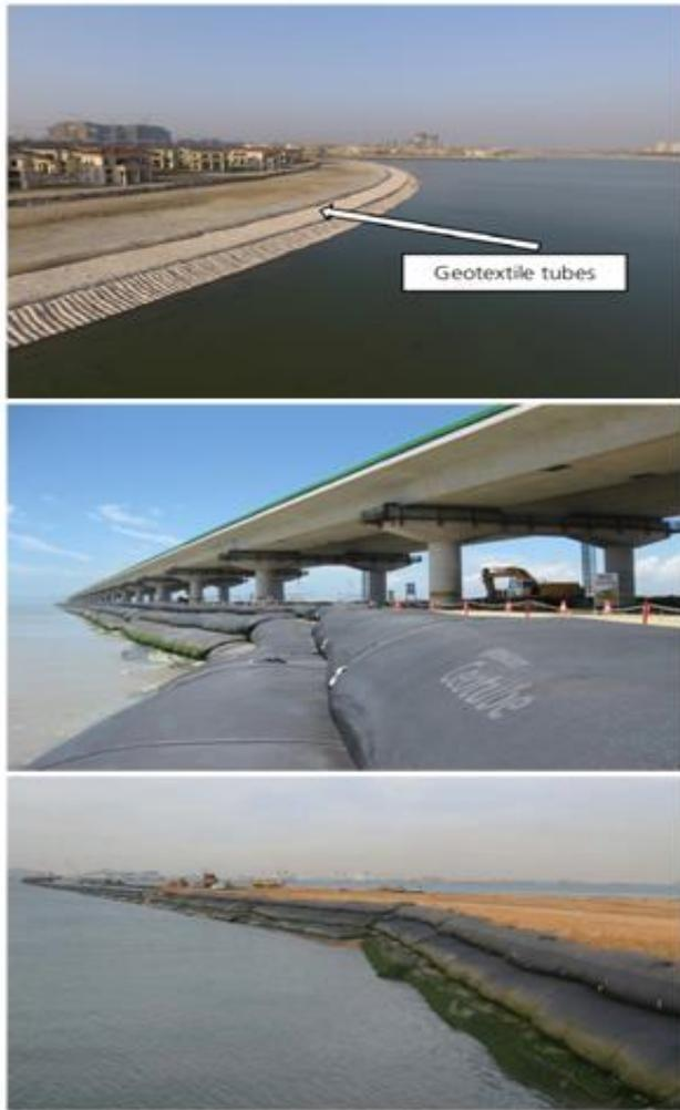
**Figure 1: Applications of geotextile tubes in several protection and storage works.**
